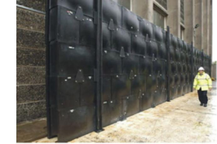
Neutron shield (water/polyethylene)
