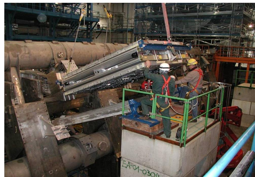
Forward Muon Spectrometer: big wheels installed, end-wall wheel installation started
