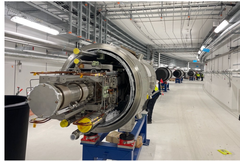
installation of SIS100 dipoles Apr'24
