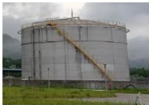
5000 m³ LAB storage tank
