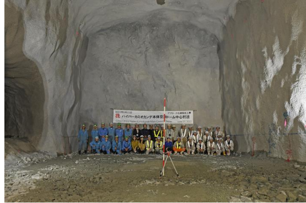
2022: Centre of the dome reached
