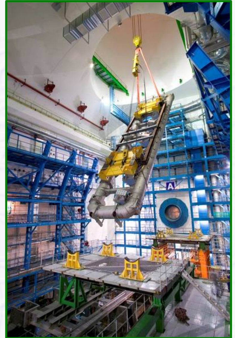
Transport and lowering of first superconducting Barrel Toroid coil
