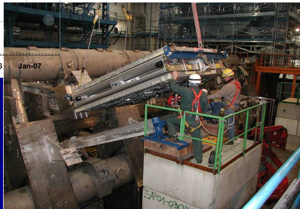
Installation of barrel muon station
