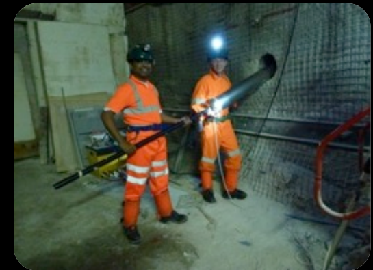
Bore hole detector installation
